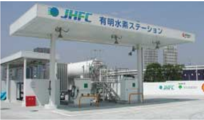
Ariake hydrogen station
