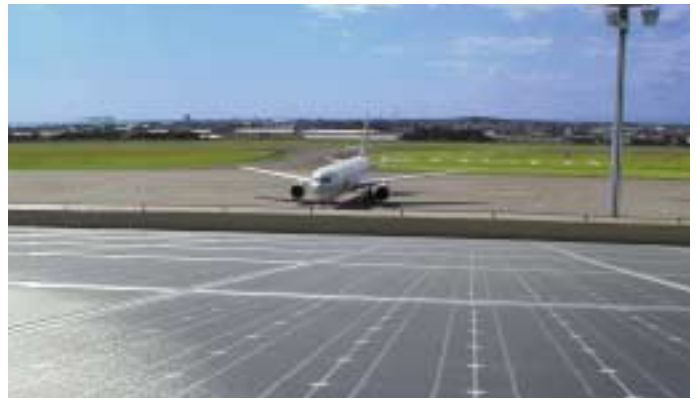
Solar power generation project at Kochi Airport
