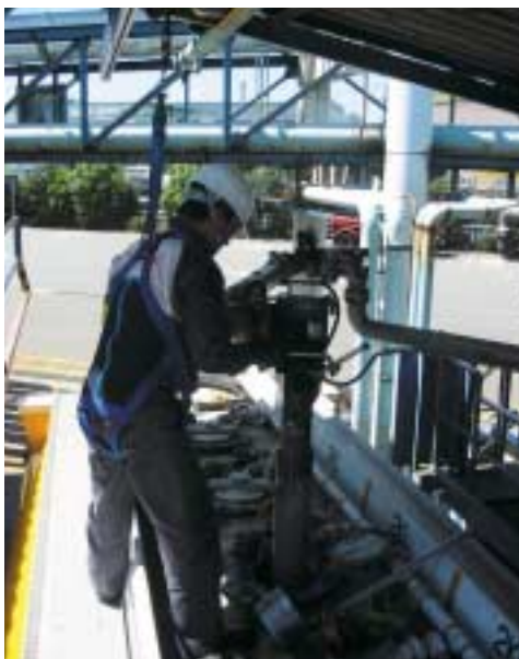
Loading operations at a refinery of the Showa Shell Group: a full harness system is being installed at each loading area of the group's refinery and depot.
