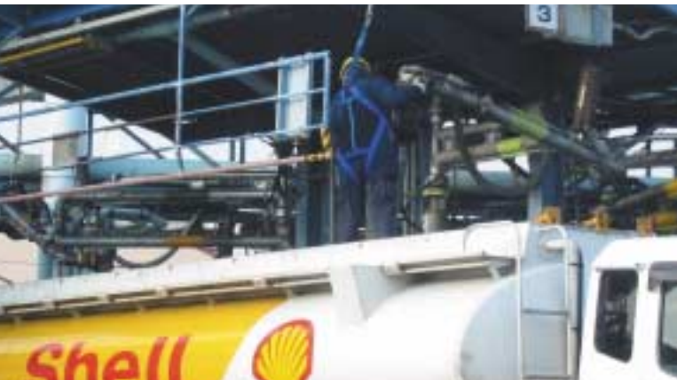
Loading operations at a refinery of the Showa Shell Group: a full harness system is being installed at each loading area of the group's refinery and depot.
