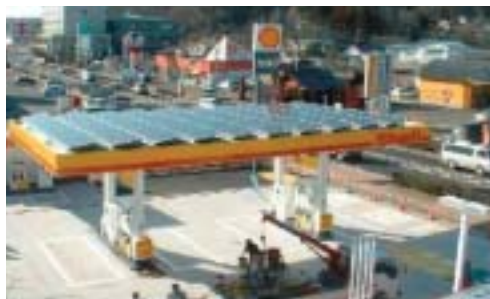
A service station with solar batteries installed.
