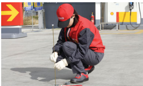
Inspections of leak detector tubes
