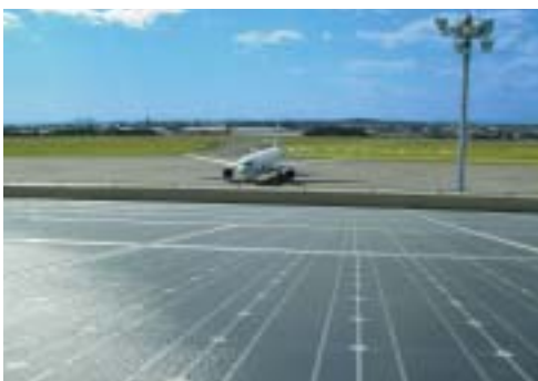
Airport installation of solar power generation system
