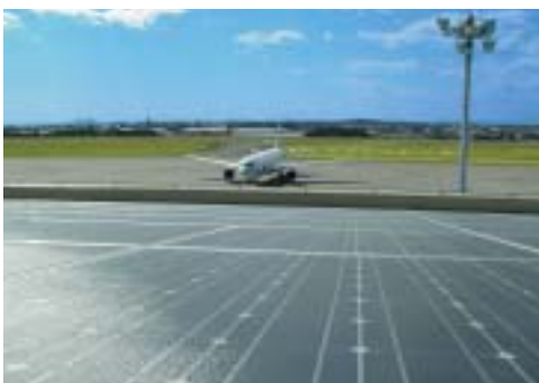
Airport installation of solar power generation system
