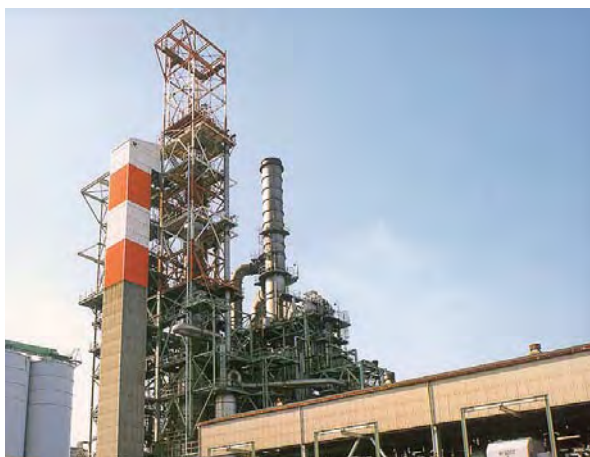
Catalytic Reformer at a group refinery
