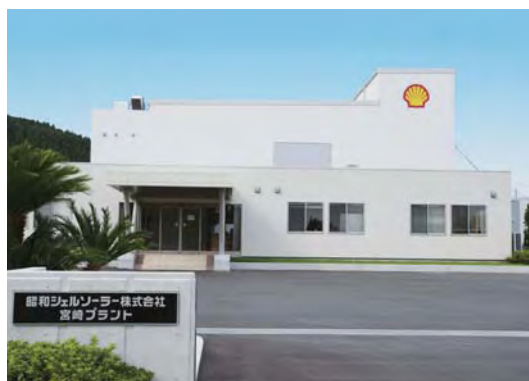
Miyazaki Plant. Commercial production of CIS solar powered cells began in 2007
