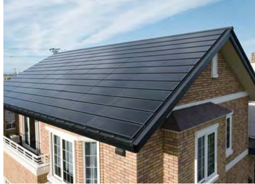
CIS solar powered cells installation example
