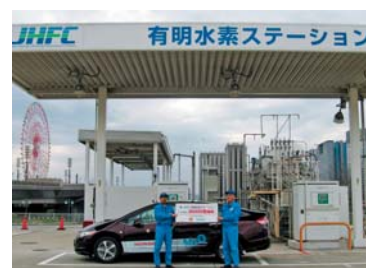
JHFC Ariake Hydrogen Station
