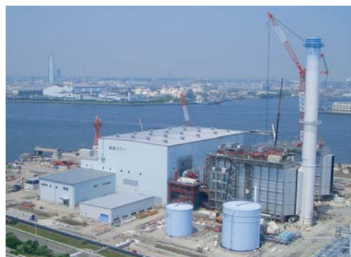
The Ohgishima Power Station under construction
