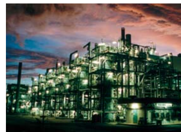
GTL plant in Malaysia
