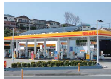
Disaster-proof service station (Fujisawa City, Kanagawa Prefecture)
